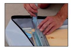
Locate the second section of counter and perform step two for the single metal leg on this counter.
