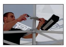
Slide the opening onto the center tent pole at a height that is above all scissor pieces.
